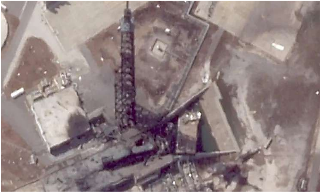
Figure 3. Post-event satellite image showing damage distribution around the launch mount and flame-trench/duct region.
